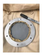
Then make holes with a sharp implement as close to the edge of the fire retardant fabric selvedge as you can to allow you to push the bolts through the canvas.
