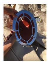
• Place one of the metal rings onto the outside wall of the tent over the stove hole and mark the position of the holes with a permanent marker.
